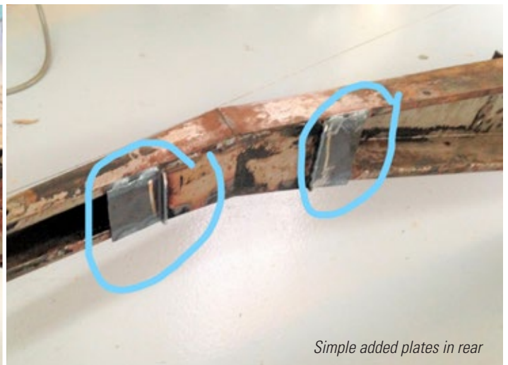
Underside of Tee gets welded
