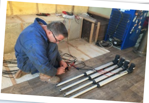
Metal guides and rams being fitted
